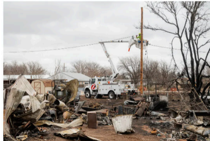
Workers replaced power lines that the Smokehouse Creek Fire damaged last month in
