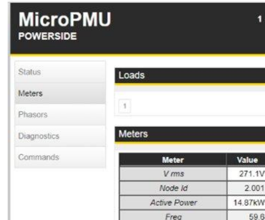
Fig. 6. μPMU data monitoring at node2
